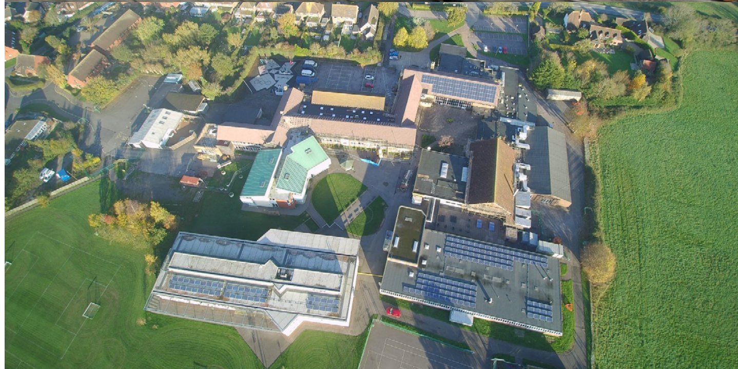
Installation on the roof of Priory School, Lewes © Andrew Aitchison
